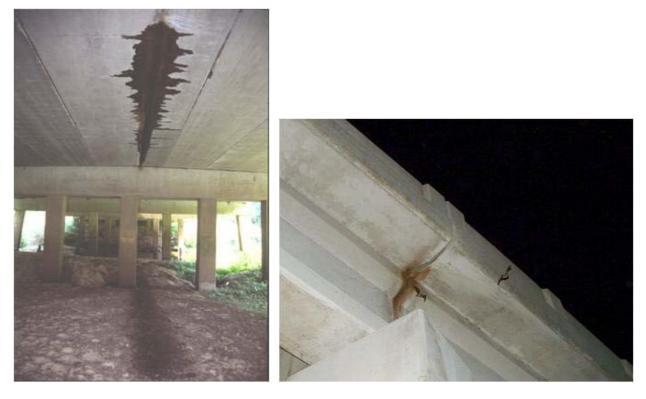
Photo 7: Staining along longitudinal joint. Note Photo 8: Staining on underside of expansion joint from bat use. guano deposits on the ground.
