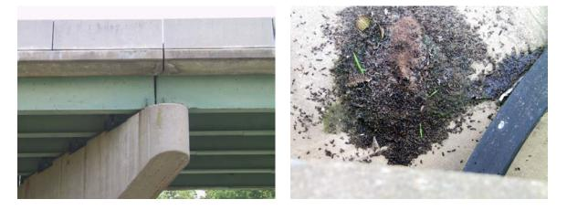
Photo 3: Example of open concrete joint used by bats Photo 4: Guano deposits visible from bridge deck, on top of pier
