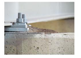
Photo 5: Guano deposit on pier, obscuring structural features.
